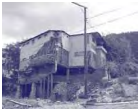
Evidence of deficient support elements for the building.
