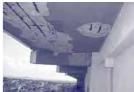
Steel exposed by loss of covering.
