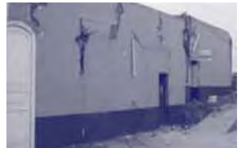
Typical failures in adobe construction.
