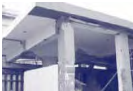
Severe damage in beam/column connection.
