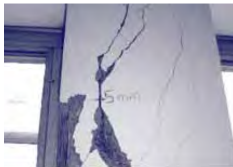
Cracks in concrete columns.
