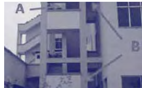
The emergency stairwell of a hospital (A), was "anchored" to the main building structure (B). In an earthquake this created a torsional response.
